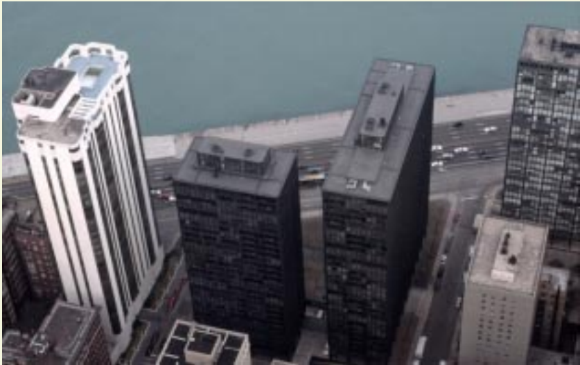
Mies van der Rohe, Esplanade Apartments , 1953-1956.
